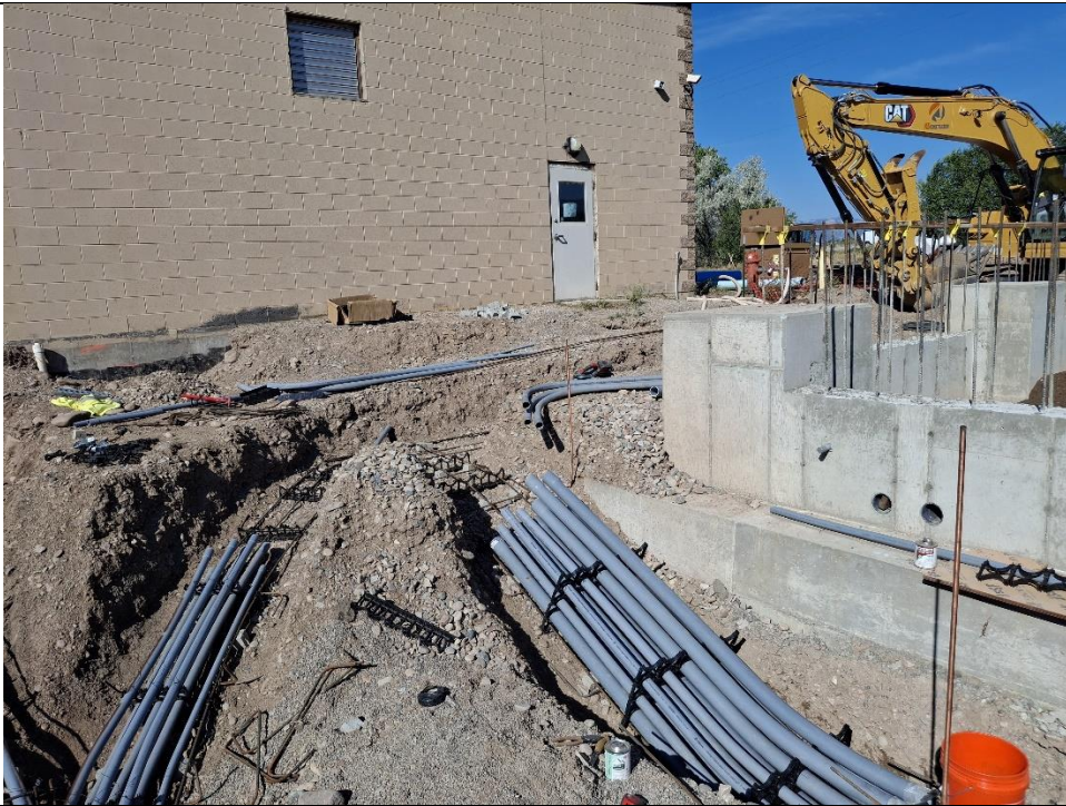
Electrical Ductbank Install
