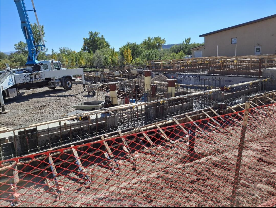
Footer Rebar & Concrete Cont.
