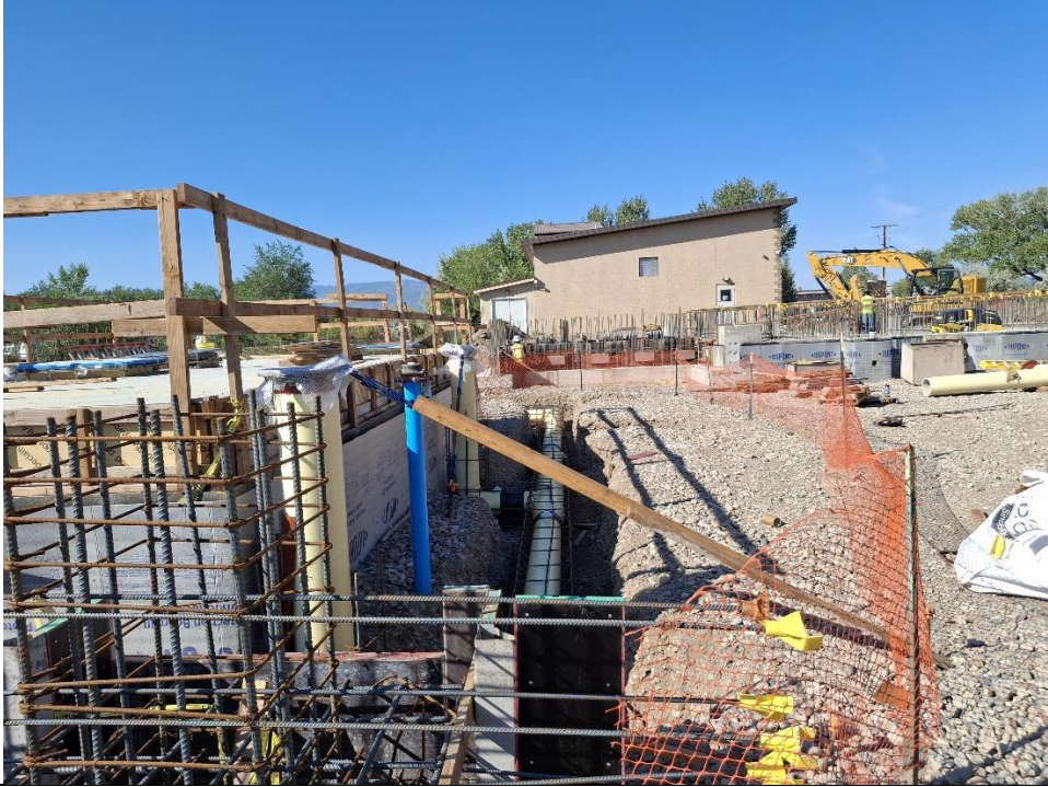
Underslab Pipe Encasement
